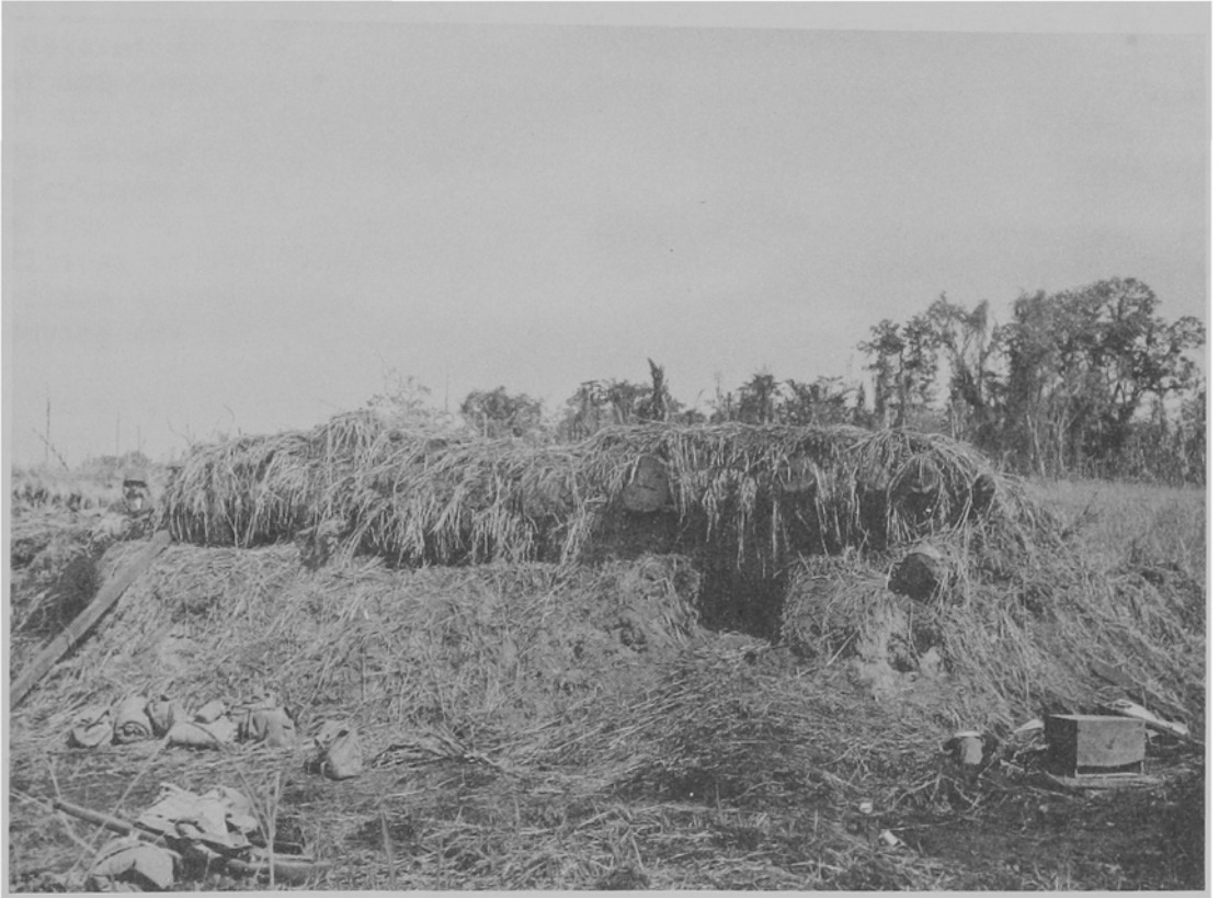
Figure 20. Buna, New Guinea: Front View of a Japanese Bunker (Pillbox).
