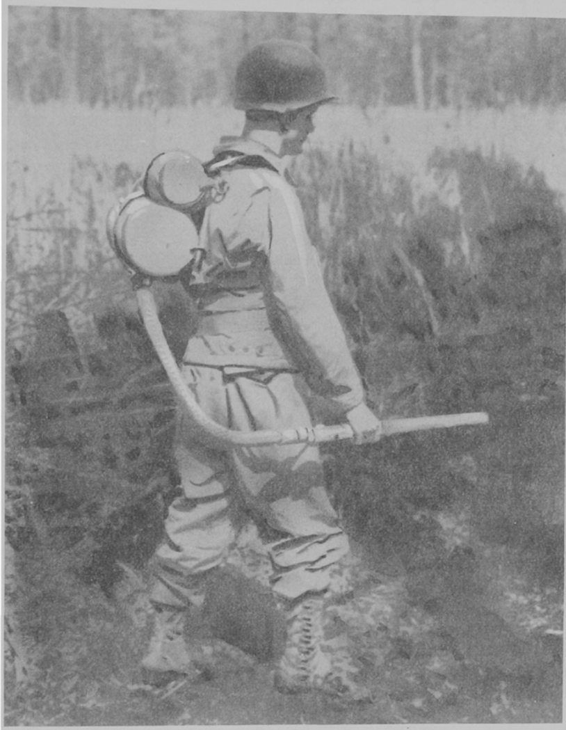
Figure 8. German Model 42 Portable Flame Thrower.
